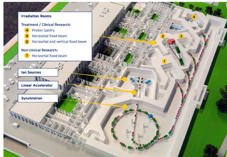
MedAustron, 25 m diameter synchrotron, 3 treatment rooms, proton gantry
